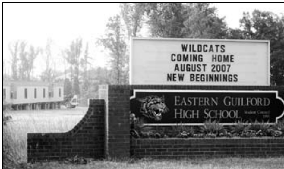
Estimated cost of replacing burned-down Eastern High School in Guilford County is $61 million but an insurance settlement is still being negotiated. (CJ photo by Sam Hieb)
