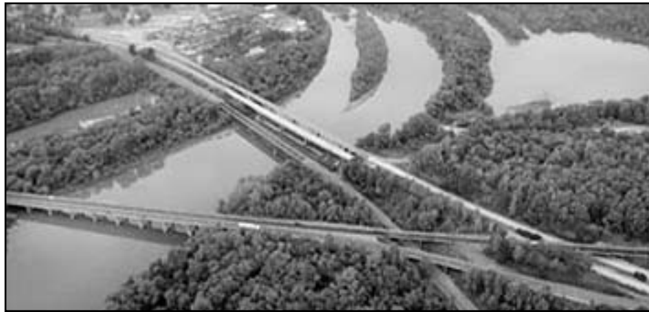
A new I-85 bridge over the Yadkin River to replace the current one (the lower bridge above) is one project being discussed. It has a $400 million price tag. (Photo courtesy Salisbury-Rowan Economic Development Commission)
