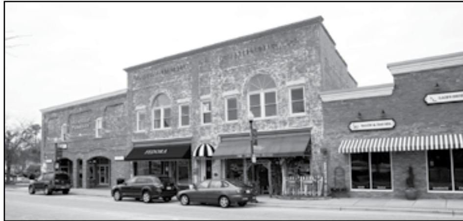
The owner of the restored Hinton & Son Hardware building in downtown Apex (center building) received a 20 percent state Historic Preservation Tax Credit. The owners of the adjacent buildings restored their properties without the tax credit. Cultural Resources Secretary Susan Kluttz featured the Hinton building on her tour to promote the restoration of the expired restoration tax credit. (CJ photo by Don Carrington)
