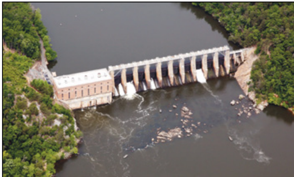
The Falls Dam area is in the segment of the Yadkin River that the state claimed was a navigable river in 1789. (CJ photo by Don Carrington)
