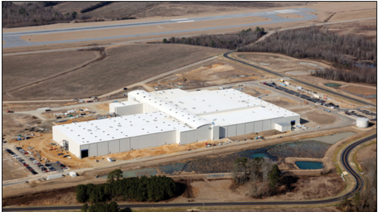
In 2008 the state landed an anchor tenant for the Global TransPark, Spirit AeroSystems, a Wichita, Kan.-based company that will manufacture aircraft components. Its TransPark facility is shown above. (CJ file photo)
