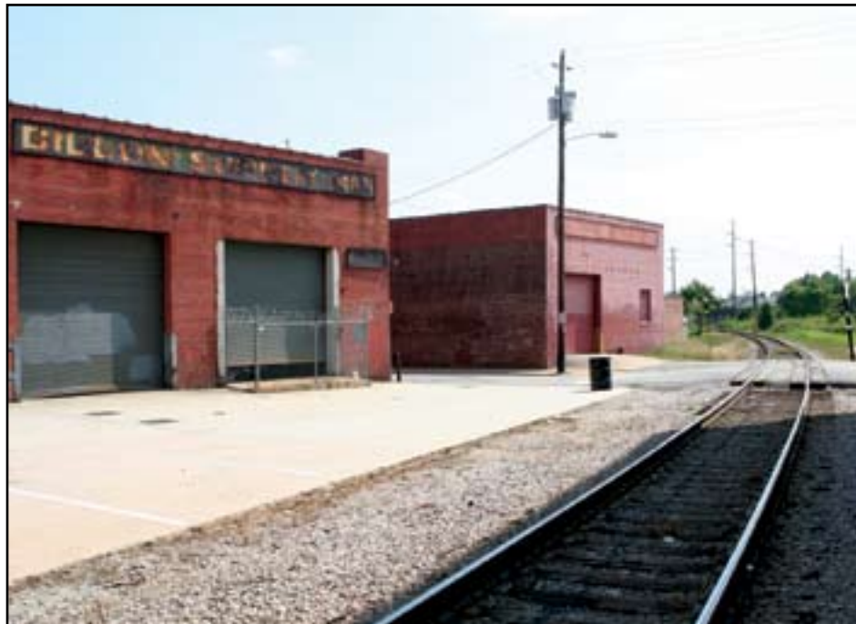
Dillon Supply in downtown Raleigh, acquired through eminent domain, is the site of what TTA hopes will be one of its 12 rail stations in the Triangle. (CJ Photo by Don Carrington)
