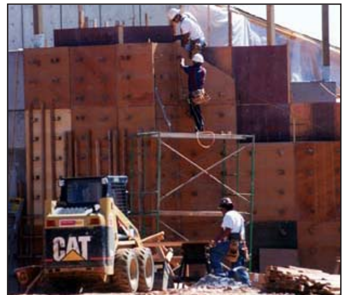
Construction on N.C. State's Raulston Arboretum.
