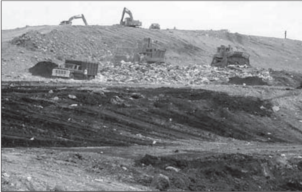
Heavy equipment at work at a landfill in Indiana.
