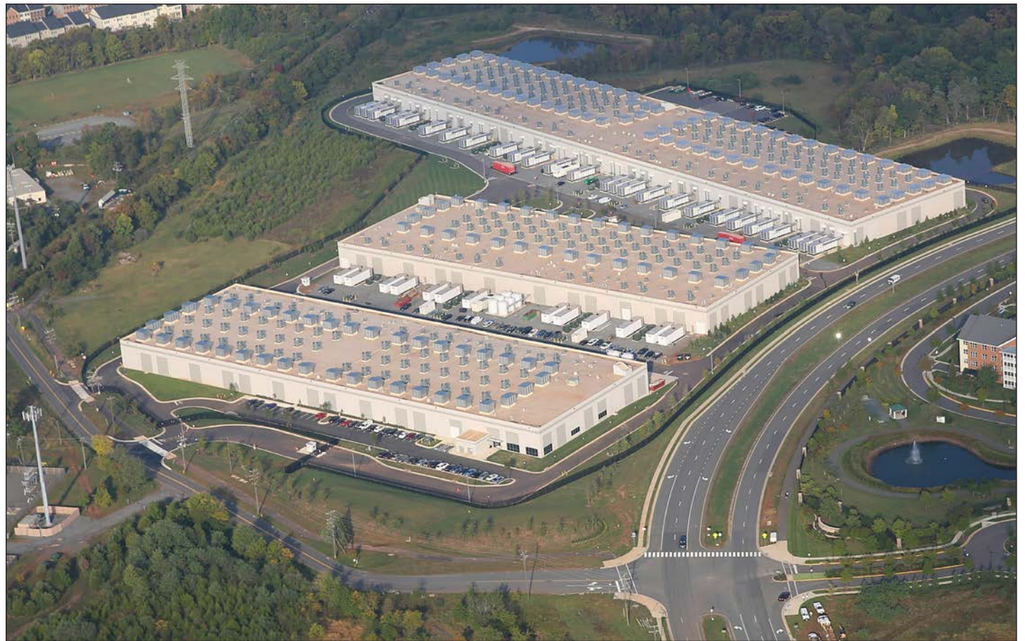
One of the Amazon Web Services data centers in northern Virginia, roughly 200 miles from the Amazon Wind Farm in Elizabeth City. (CJ photo by Don Carrington)
