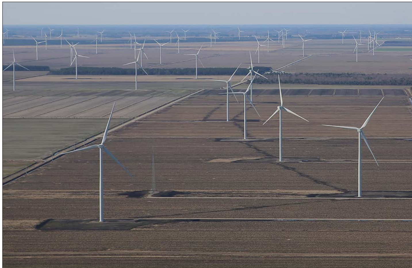
The Amazon Wind Farm, the state’s first large-scale commercial wind-generation project, comprises 104 2-megawatt wind turbines each nearly 500 feet high. (CJ photo by Don Carrington)
