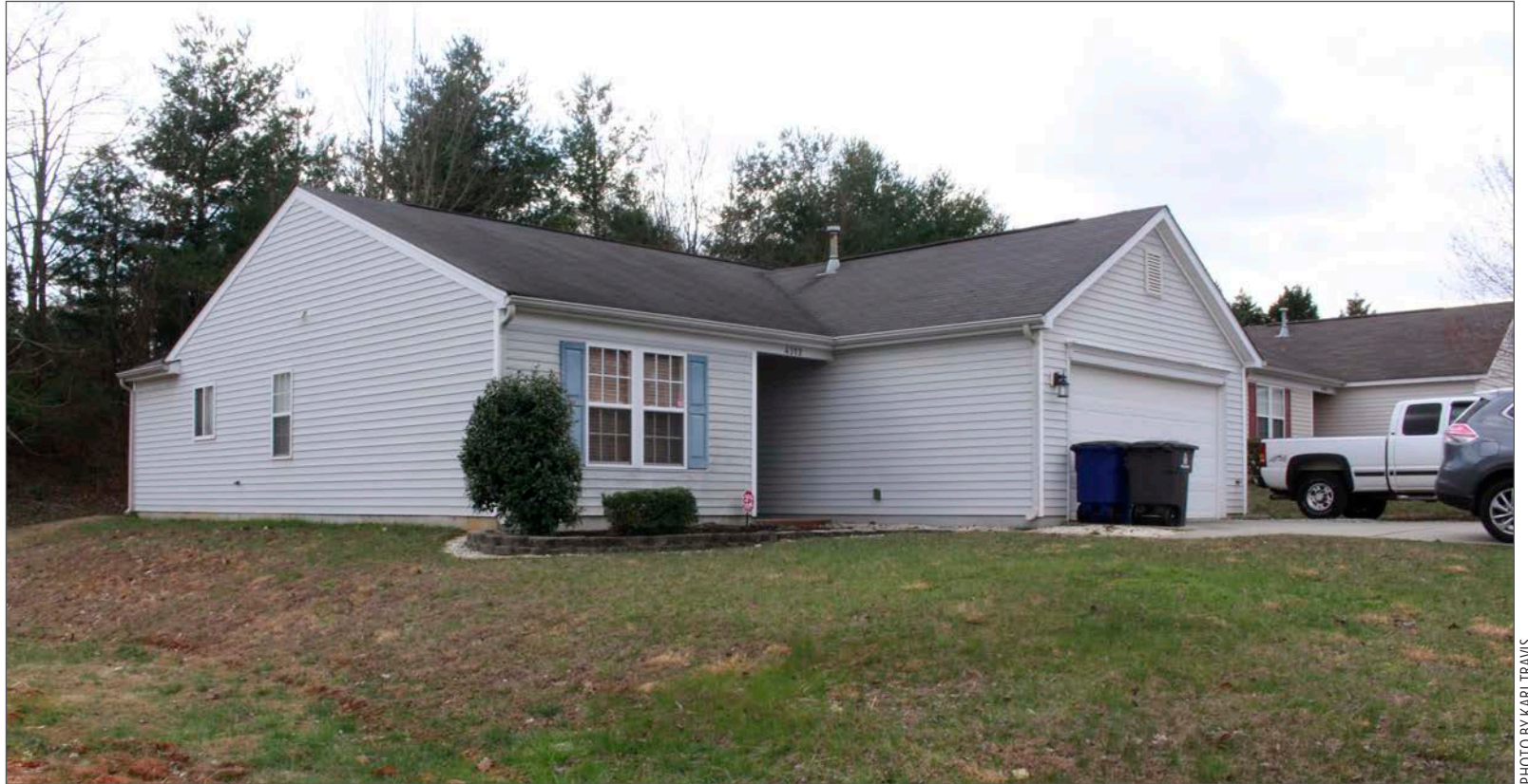
TARGETED FOR A BREAK-IN. Earlier this year, the Weeks house was broken into, which the family blames on the declining neighborhood.
